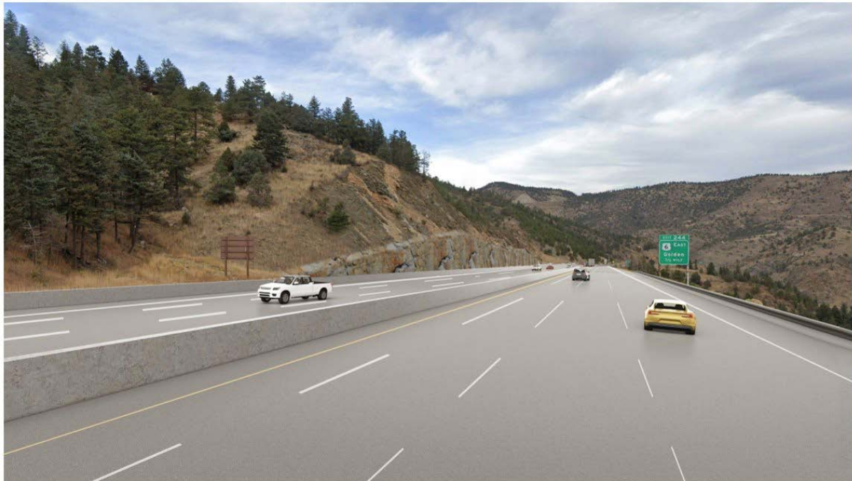
I-70 Floyd Hill to Veterans Memorial Tunnel Close up of Retaining Wall E-10 (After Improvements) - Shotcrete
