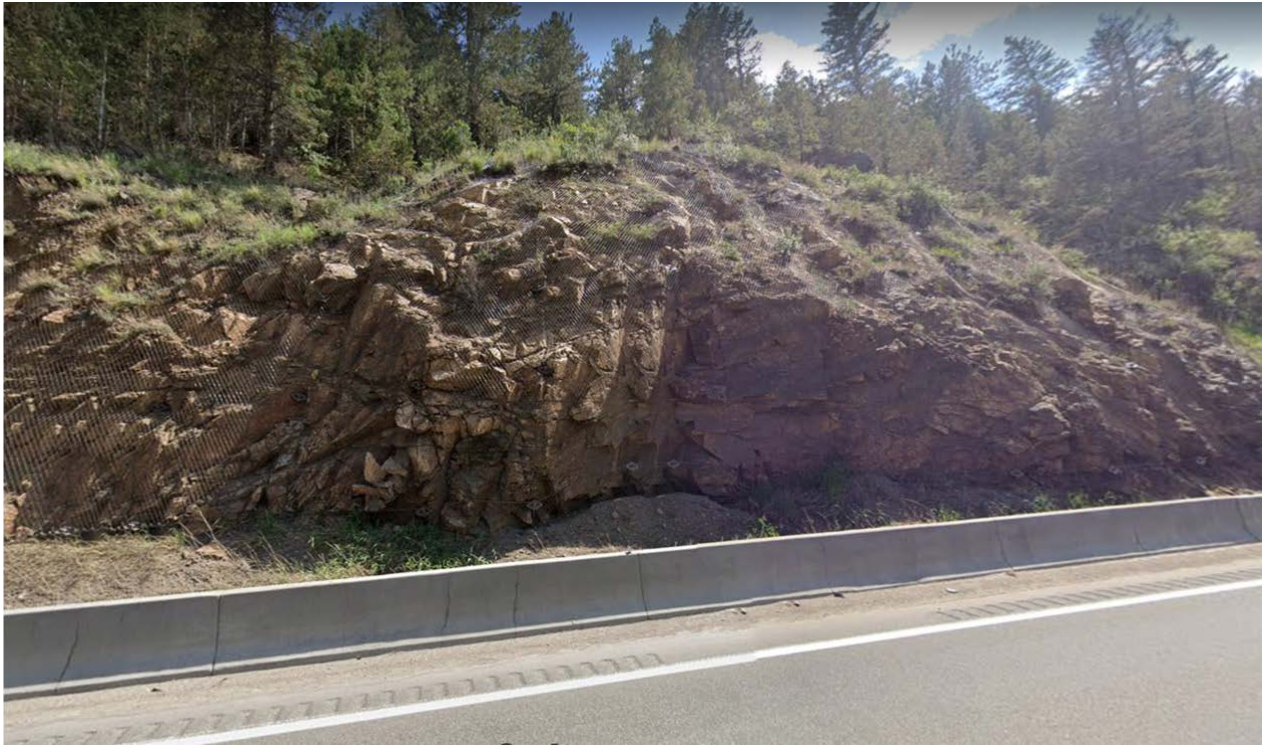
Example of how mesh blends in with a Sculpted Shotcrete wall.
